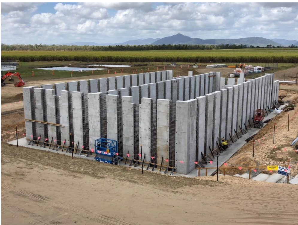
Photo 5: Erected panels at the Mirani WRF
