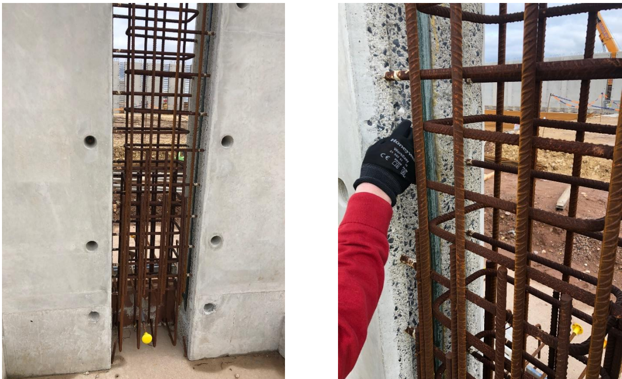
Photo 3: Semi-cast in-situ joint
