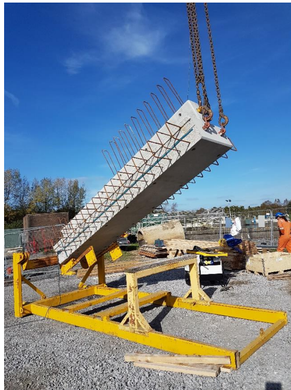
Photo 2: Semi-cast lifting device
